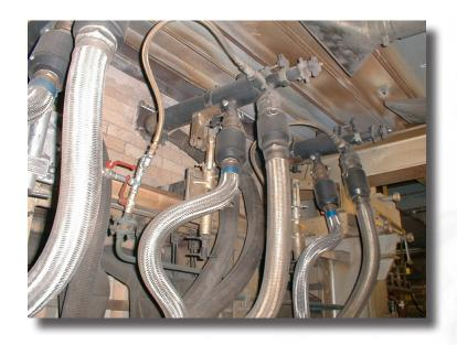
The pictures to the left showing the installation of three(3) oxy-fuel burner on an end fired furnace during a regenerator (cold) repair. All burners have fully flexible flame adjustment.
