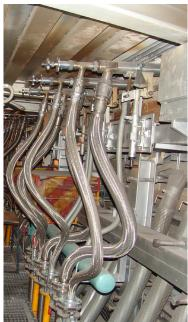
Hotwork International know-how and technology allows the replacement of conventional air-fuel burners with our specially designed oxy-fuel underport burner to replace combustion air partly or completly.
